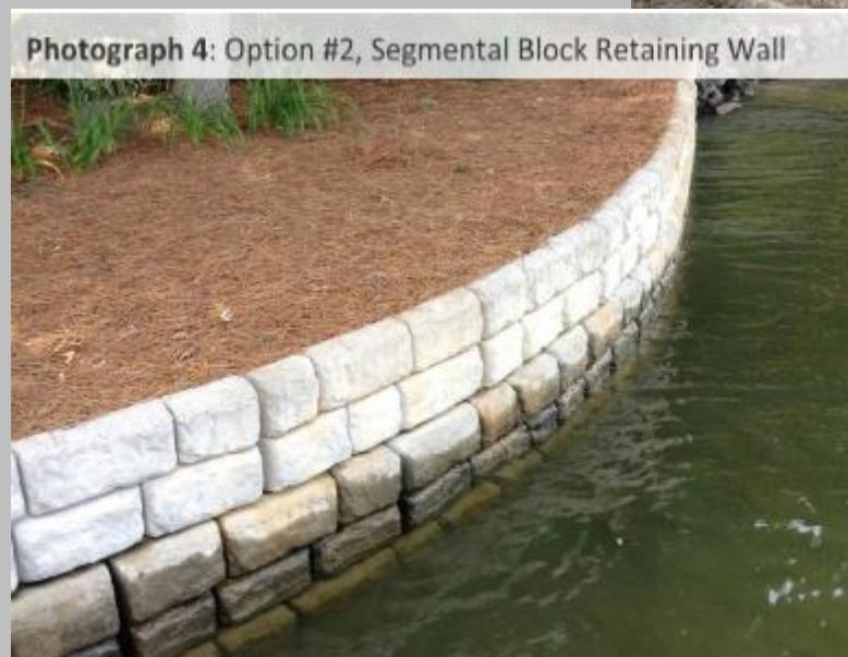
Photograph 4: Option #2, Segmental Block Retaining Wall
