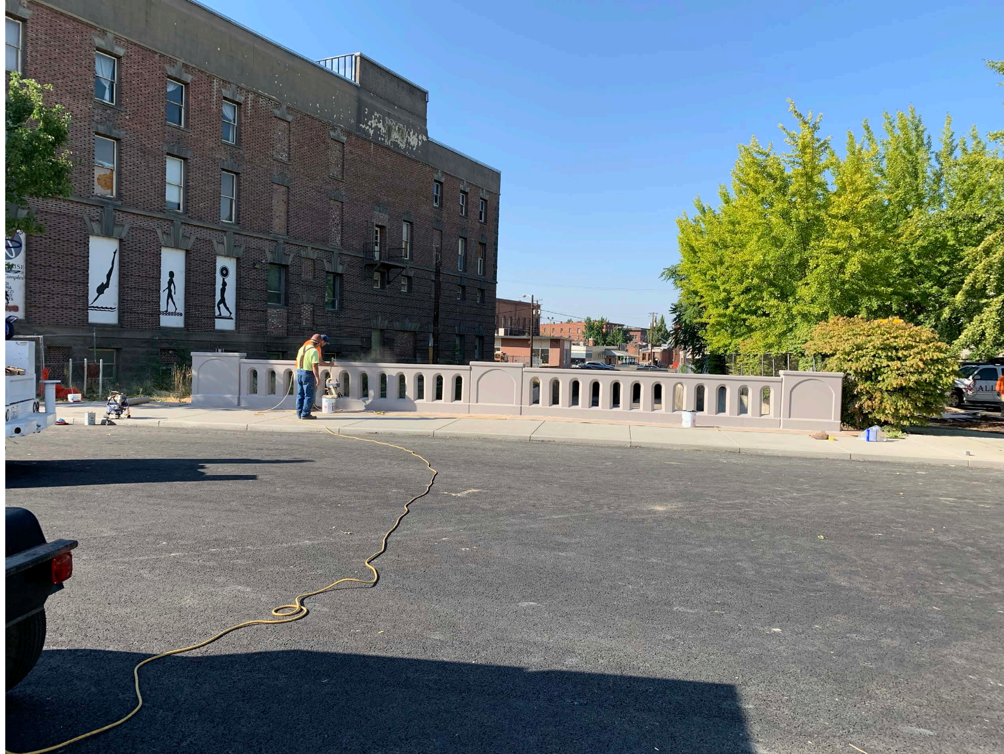
Friendship Bridge - facing west
